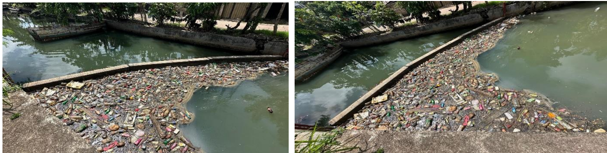
Figure 1&2: The waste is stopped by the Ocean Strainer, before cleaning the waste by Negombo Municipal Council
