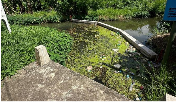
Figure 3: The waste being intercepted by the Ocean Strainer at NARA Canal and stopped floating to the Lagoon
